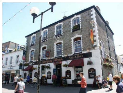
The Newquay Arms. Coursed killas rubble and granite quoins
