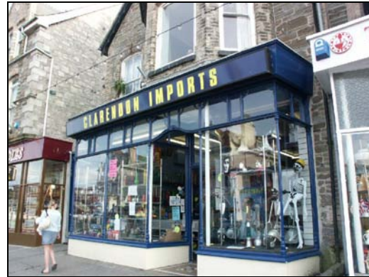
Surviving historic shop front, East Street
