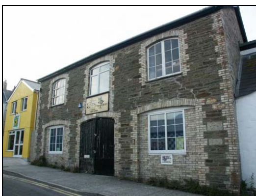
Industrial workshop, Wesley Yard. Active street frontage encloses an internal open courtyard
