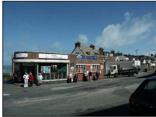
East Street bus station. There are regeneration proposals for the creation of a town square following the relocation of the bus station
