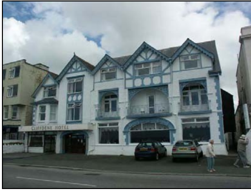
Cliffdene Hotel; a relatively domestic scaled building
