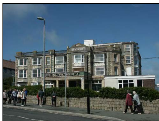
The Beachcroft Hotel: an historically significant building suitable for reuse
