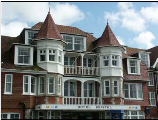
Detail of the balconies and twin turrets of the Hotel Bristol
