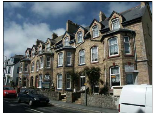
Typical Edwardian terrace, three storeys with gabled dormers, projecting bays and enclosed front gardens
