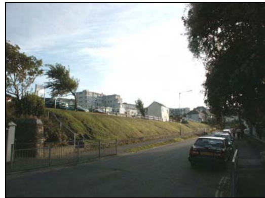
St Michael's Road, view south west. The sloping topography of Mount Wise is a significant feature of both car parks proposed for development
