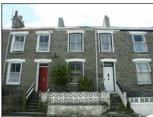
Mid – late 19 th century terraces, of slatey grey killas laid as elongated irregular rubble. The streetscape includes double and single fronted facades
