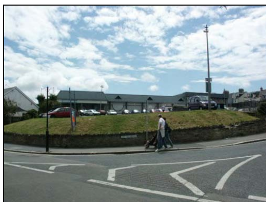
The Whim. Demolition of terraces has led to a loss of streetscape enclosure
