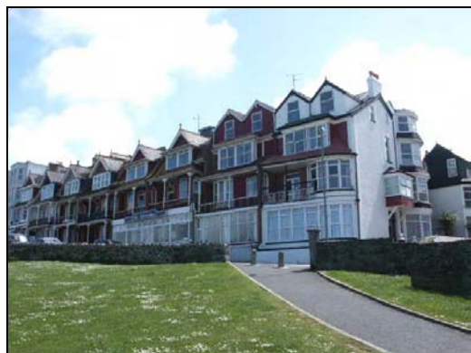
Island Crescent, shown in early stages of construction on the second edition OS map of c1907
