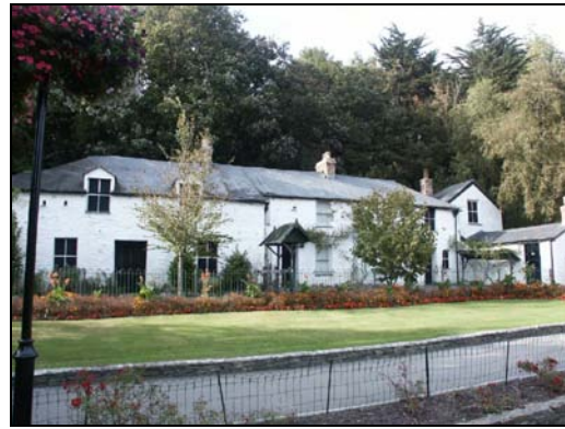
'Heritage cottages' in need of conservation and reuse
