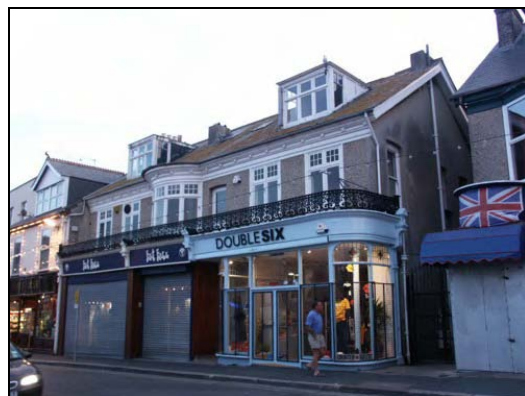
Transitional character; smaller scaled buildings retain high levels of architectural detail. Survival of historic shop fronts, cast iron balconies and oriel window are notable features.
