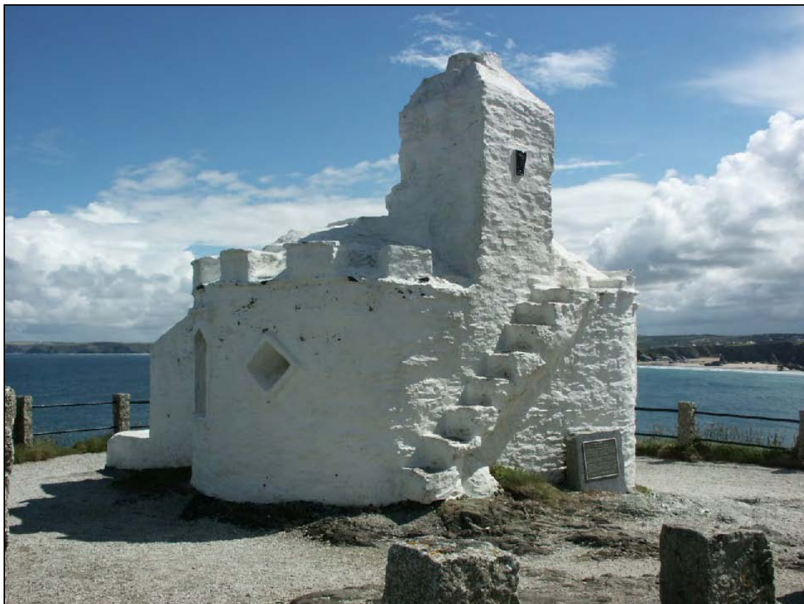
The huer's hut (Listed Grade II*). One of the few surviving structures relating to the pilchard industry.
