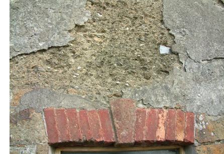
A cob wall with 'shilf' visible (small pieces of slate). The surface has partially disintegrated.
