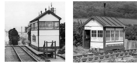
Typical GWR signal boxes, of all timber or timber and masonry construction, with similar fenestration patterns and often slate roofs.
