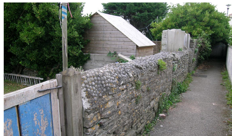
A garden lane giving rear access to houses on both sides. A killas rubble wall is capped with seashells set in mortar.
