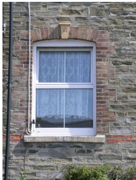
Brick quoins and arched window head with a granite sill set in a killas wall with orthogonal pointing.
