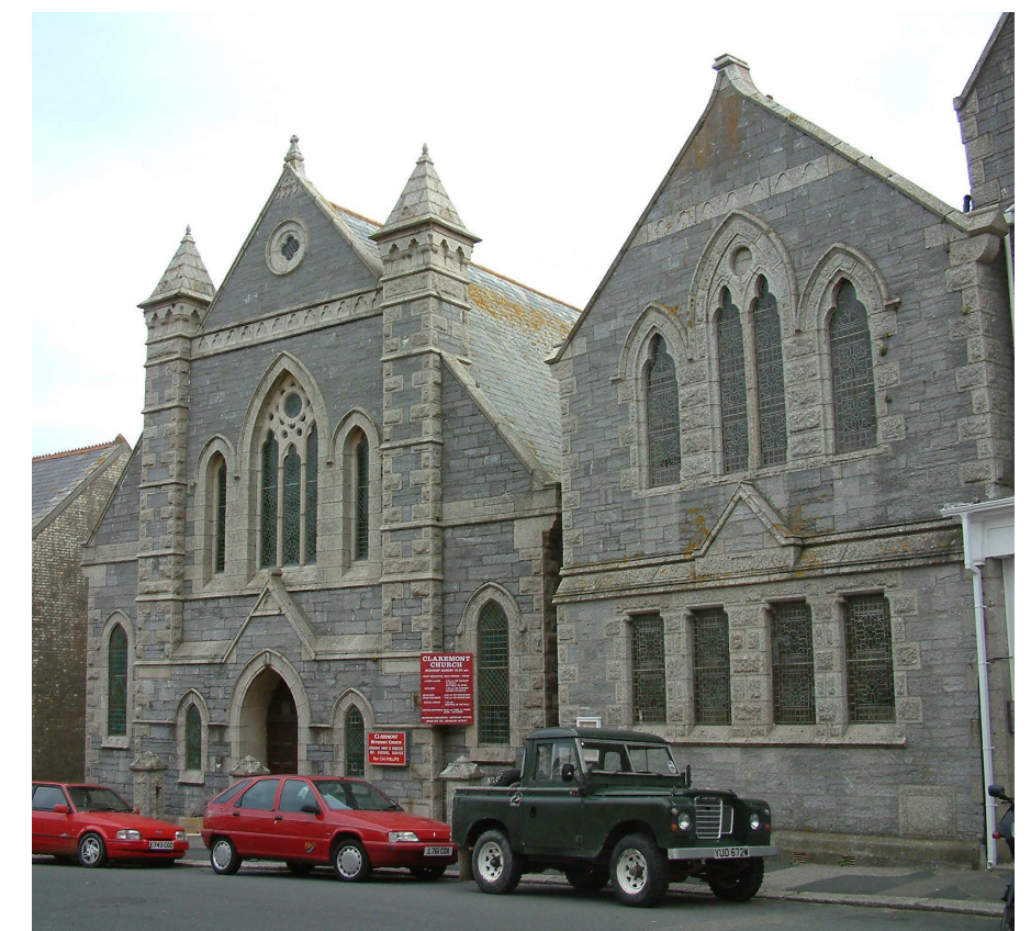
Coursed random rubble walls with granite dressings and rock-faced quoins. Massive construction common to public buildings.
