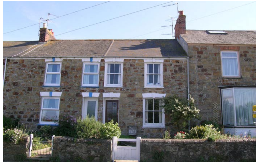
A row of cottages built from with partially squared sandstone rubble, a common technique, giving a warm, mottled effect.
