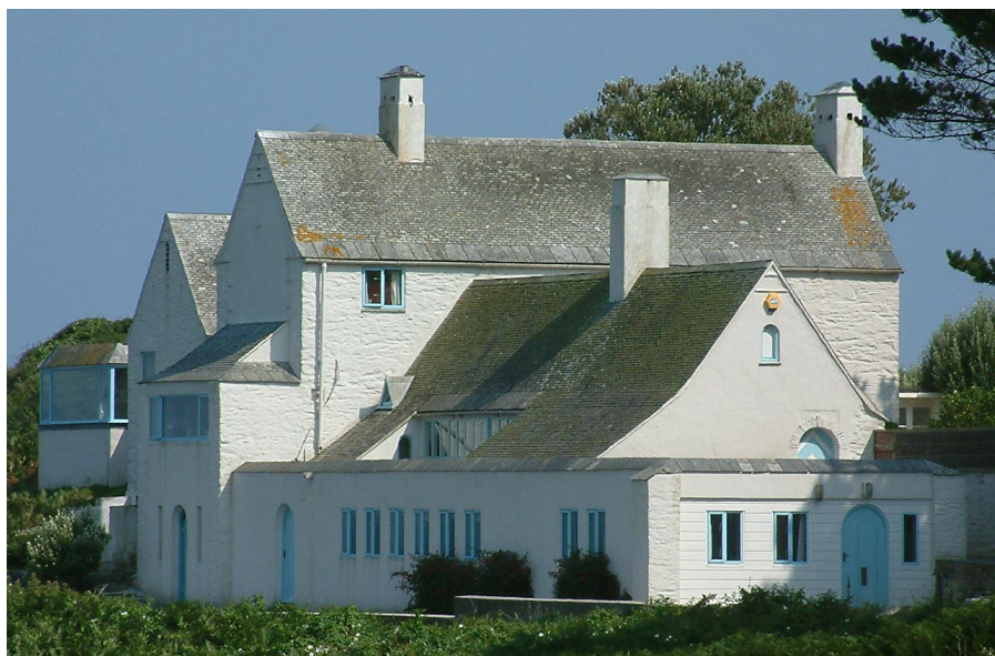
Walls of white painted random rubble with well laid slate roof.
