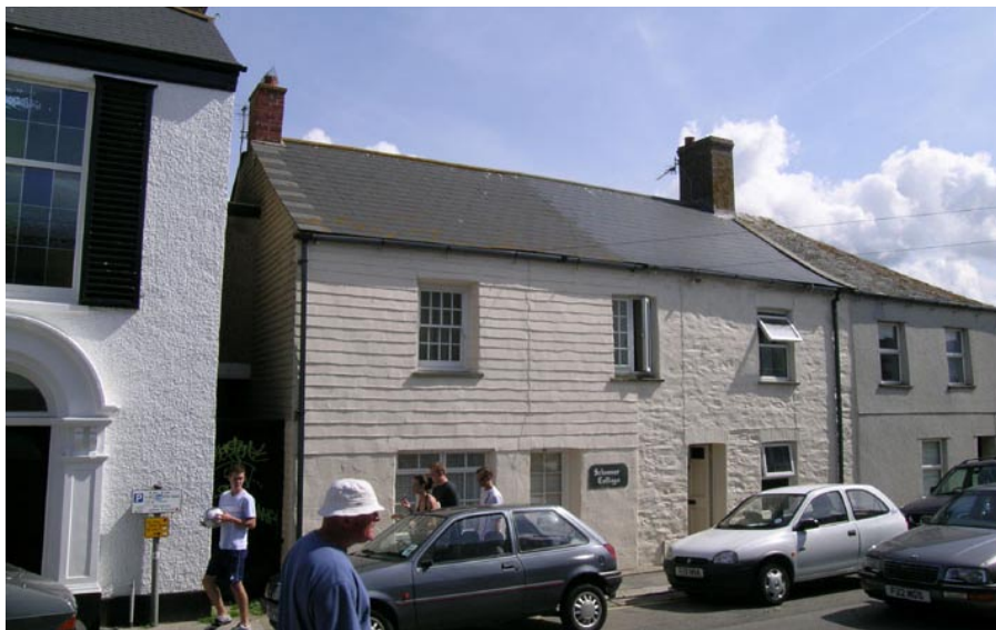
A rendered surface given the appearance of weatherboarding, a technique repeated elsewhere in the area.
