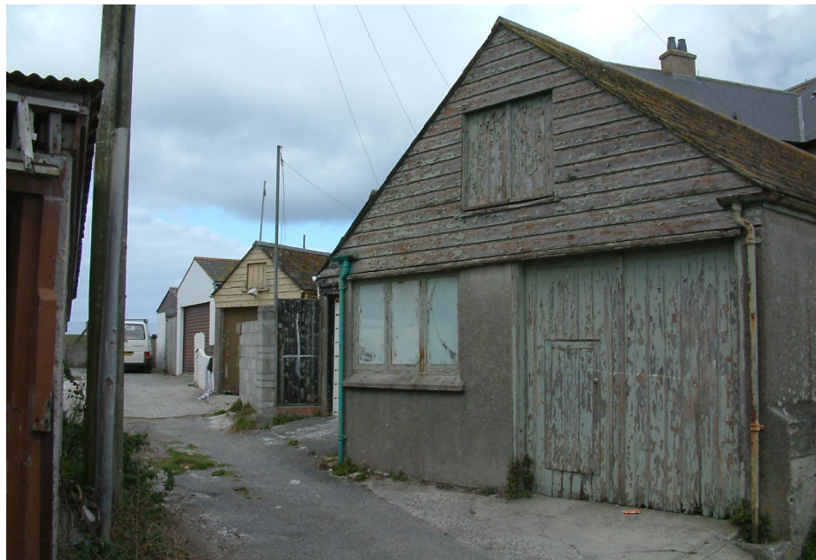
Backcourt garages. Pebbledashed walls. Horizontal weatherboarding to the gable with access hatch inset. Slate roof. Cast iron ogee gutters
