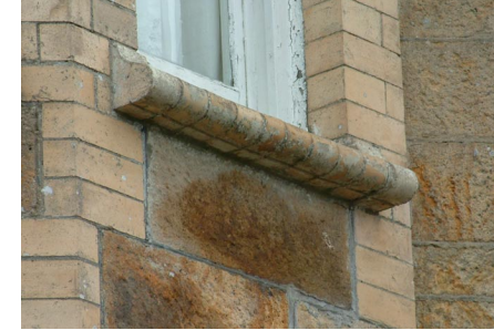
Squared sandstone wall with brick dressings.
