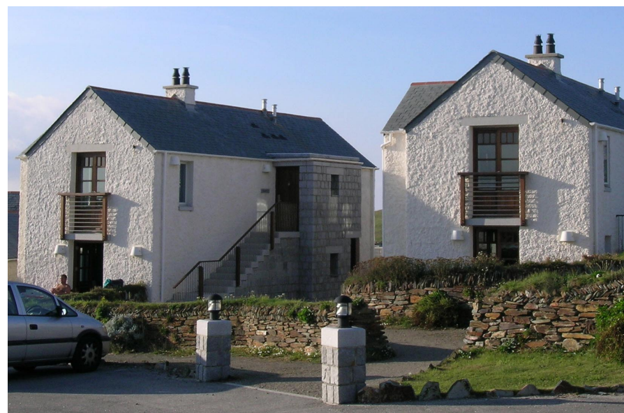
A successful contemporary application of textured render used with synthetic slates. Stone hedges help 'ground' the buildings.
