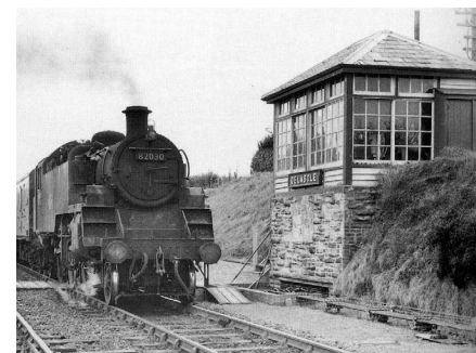
A signal box with a rubble stone plinth.
