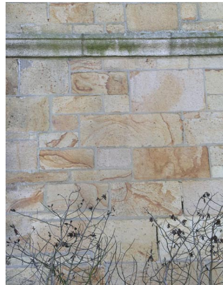
Attractive veining in a smooth-faced sandstone, squared rubble wall. The greater finish is appropriate to a church or public building.
