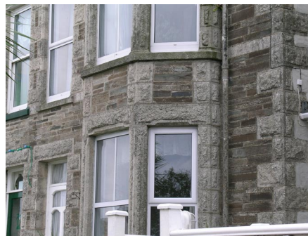
A killas squared rubble wall with rock-faced granite dressings that have chisel-drafted margins.
