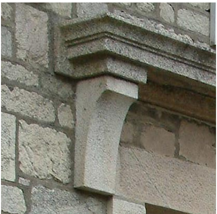
Granite corbel and hood moulding above the main entrance, Crantock Street.
