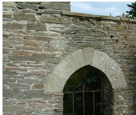
Granite voussoirs set in a killas rubble wall, the larger stones are used for the higher section of wall.
