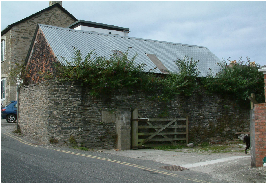
Brick workshop with a corrugated iron roof, enclosed by a slate-stone rubble wall.
