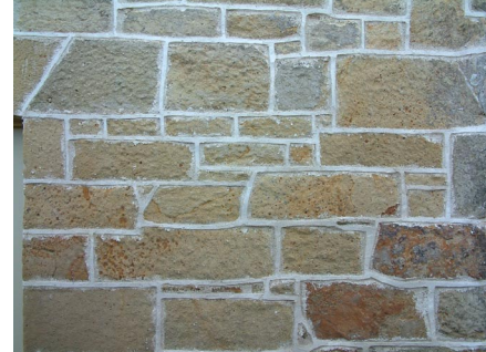
Sandstone partially-squared rubble walls.
