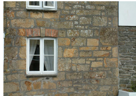
Sandstone partially-squared rubble walls.
