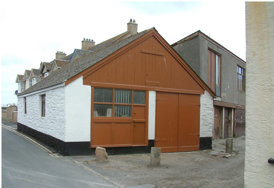
Garage at the entrance to a Backcourt with limewashed rubble walls, timber doors, a boarded gable with access hatch. Corrugated roofing with eaves kept close to the walls
