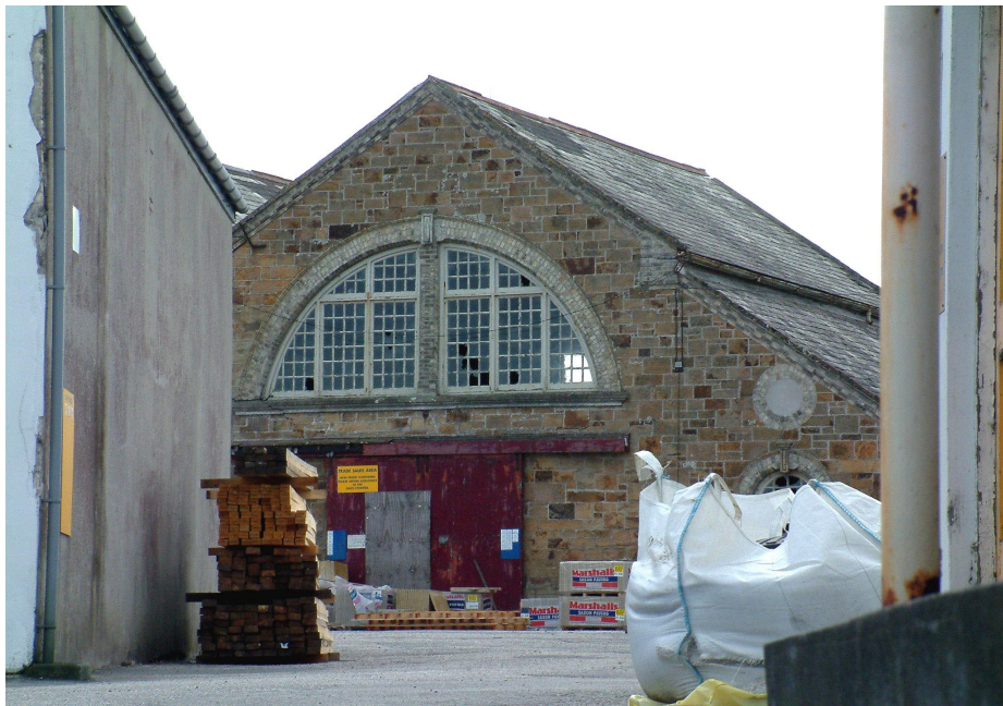
Sandstone factory building with thermal window and brick dressings
