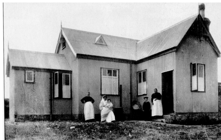
Corrugated iron or "crinckly tin", arguably a local material, here used for both roof and walls of a community building.
