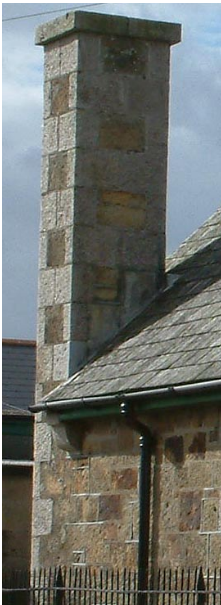
Hope Terrace- chimney with granite quoins and cap.
