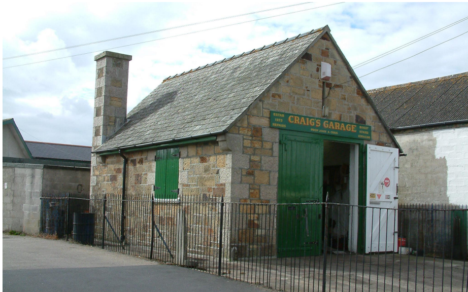
Hope Terrace- a simple and robust garage. Sandstone squared rubble with granite dressings. Framed, ledged and braced matchboarded doors.
