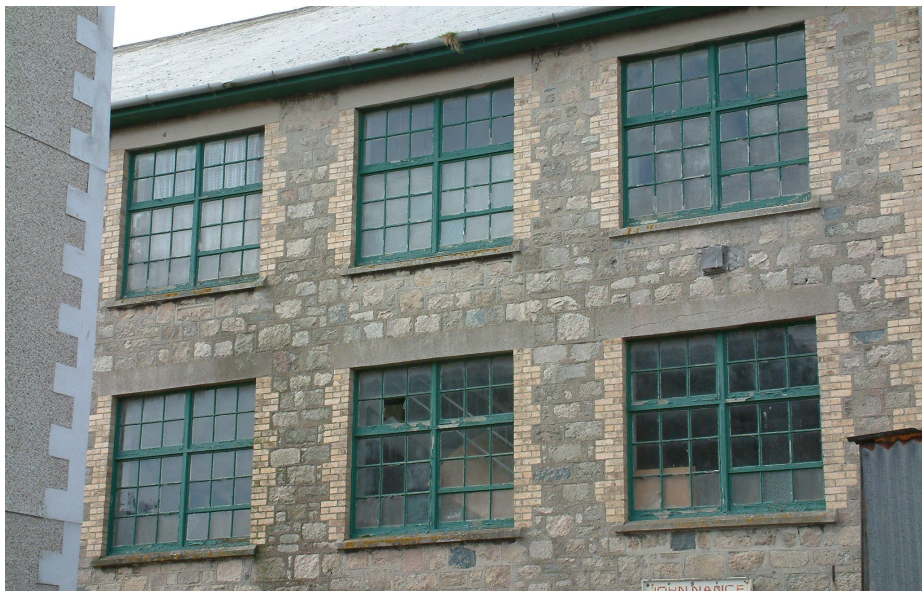
Crantock Street- large windows on a side elevation. Rubble wall with brick dressings.
